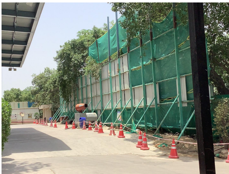
Fig. 4: Photograph Showing Barricading at the Project Site
