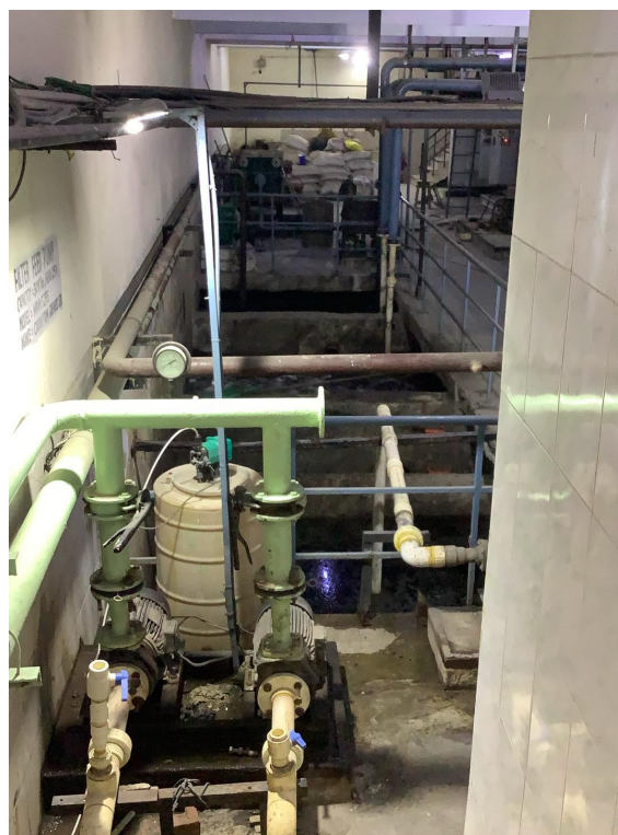
Fig 3. STP installed with capacity of 600 KLD
