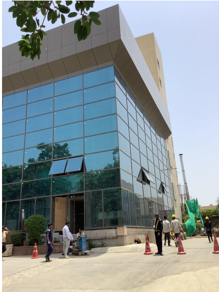
Fig. 1: Site Photograph Showing the Project Building
